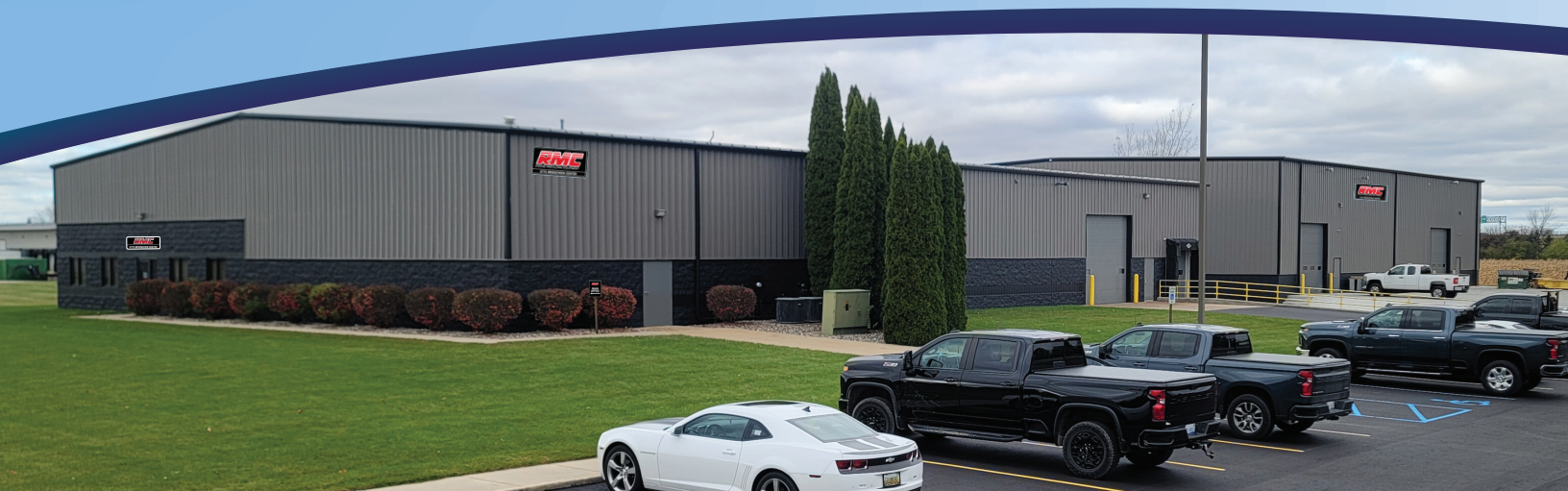
Original Saginaw Facility built in 2000, 15,000 SF
